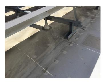
Examples of damage to a TPO roof from solar arrays.
